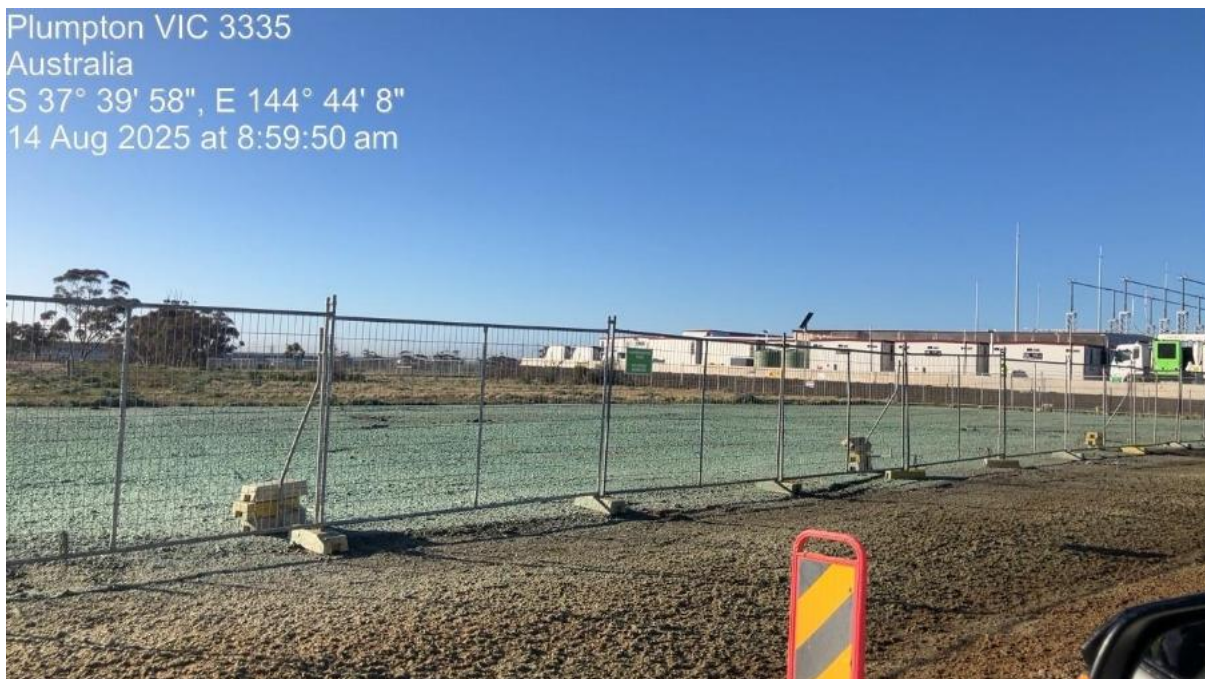
Photo 1 -Taken by Contractor -Temporarily disturbed area following hydroseeding
